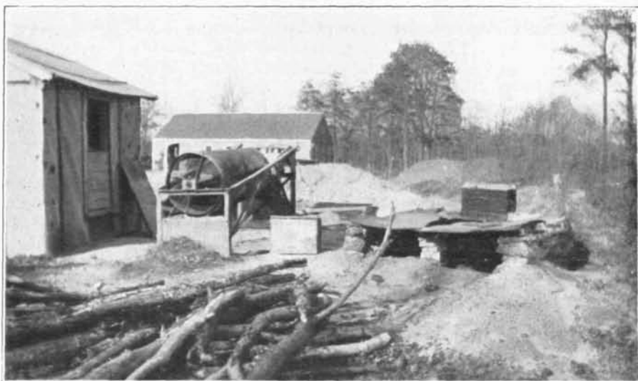
Soil-baking oven for killing weed seeds.
