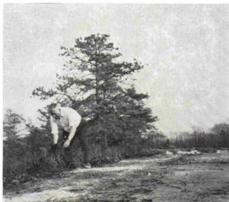
Eb Steineger raising a "blanket" of vegetation lifted from adjacent areas to cover slopes of the new tee, giving it that "natural look."
