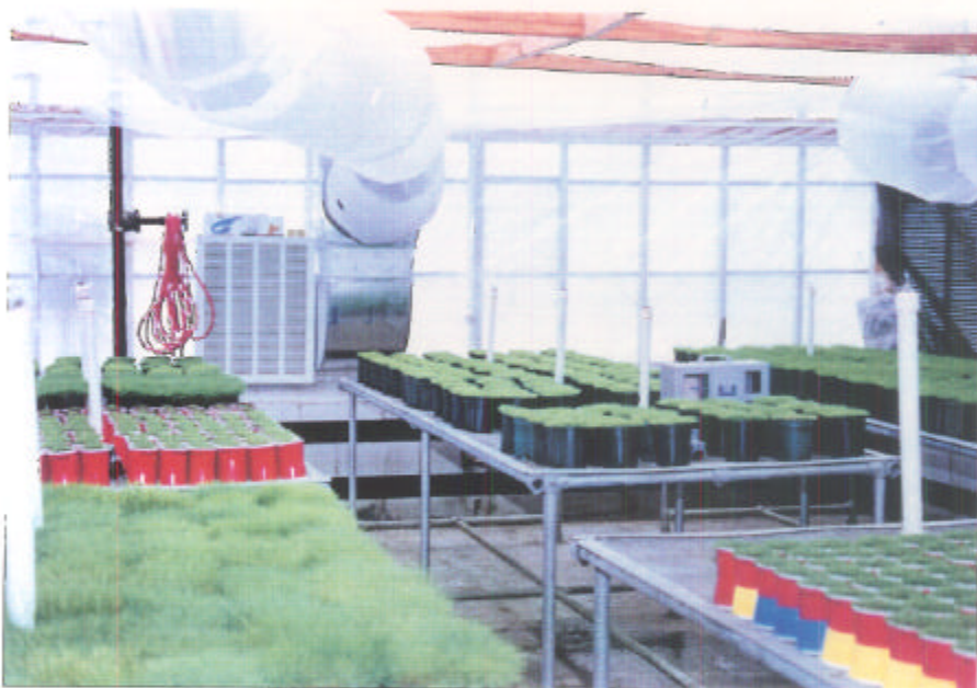
Figure 3. Inside the environmental control greenhouse bentgrass variants are maintained at 17°C. The plastic convection tubing suspended from the rafters serves as the duct work, providing optimum air circulation.
